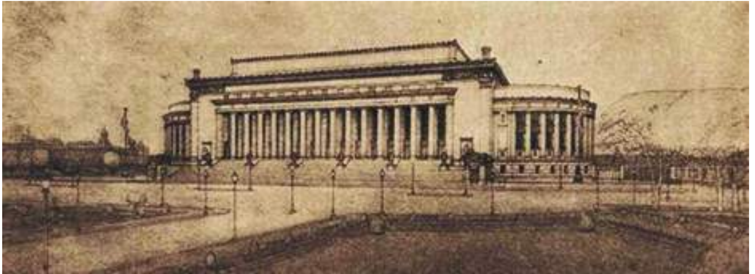
Figure 20: Post Office Building, Manila, built 1926
